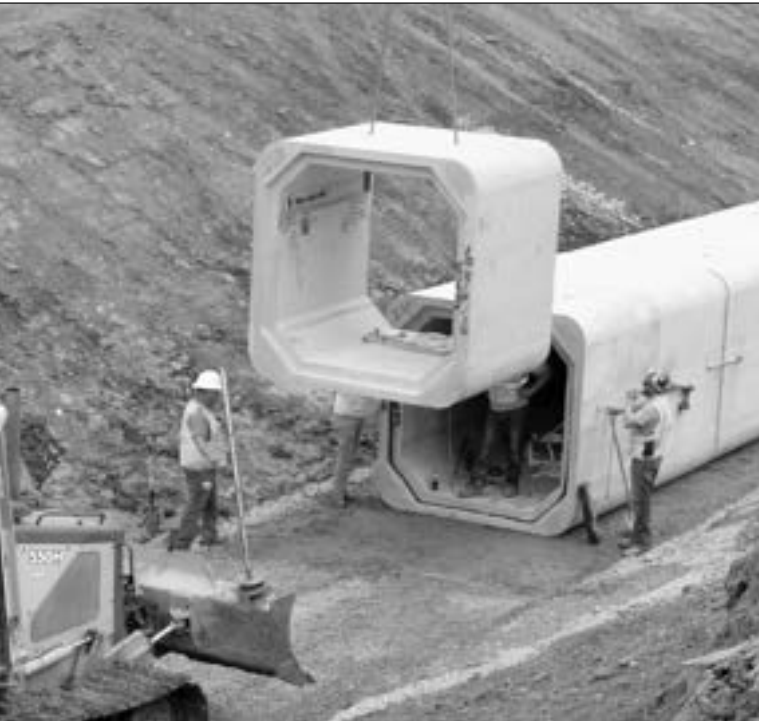
NEW CULVERT - Almost 170 feet of culvert with an interior diameter of six feet were laid at the south end of Waseca County 23 in Wilton township to replace an aging culvert installed in the 1940s. More than 20 pre-cast concrete pieces form the waterway were set 17 feet below the level of the roadbed using a crane capable of extending more than 200 feet. Star Eagle photos by Deb Bently
