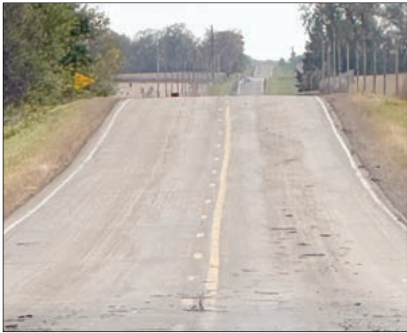
VISUAL TRAP - This roadway in Waseca County provides an example of a "visual trap." An unfamiliar driver could easily believe this road continues straight ahead, but the hill is concealing a curve.
