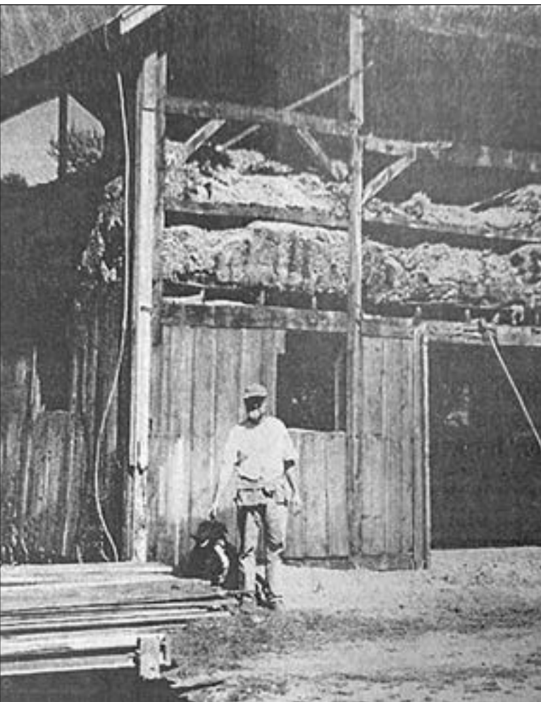
- Each board of the barn on the Verna Schoenrock farm built in 1923 is being carefully removed by Richard Jefferies. Richard has been dismantling barns for nearly 25 years. The salvaged materials are used in a number of ways.
