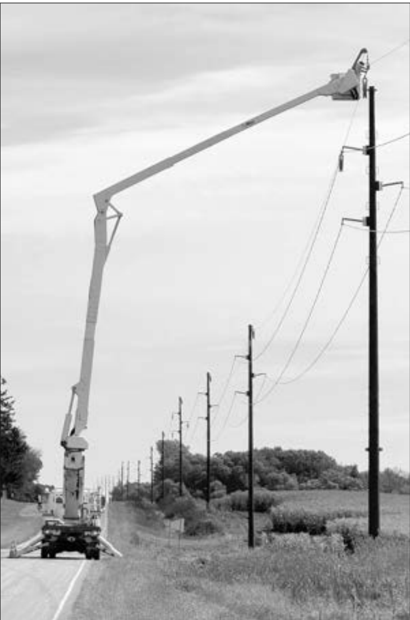
Crews working for Great River Energy began removing wooden posts last spring, a project which will now be completed in November instead of October.
