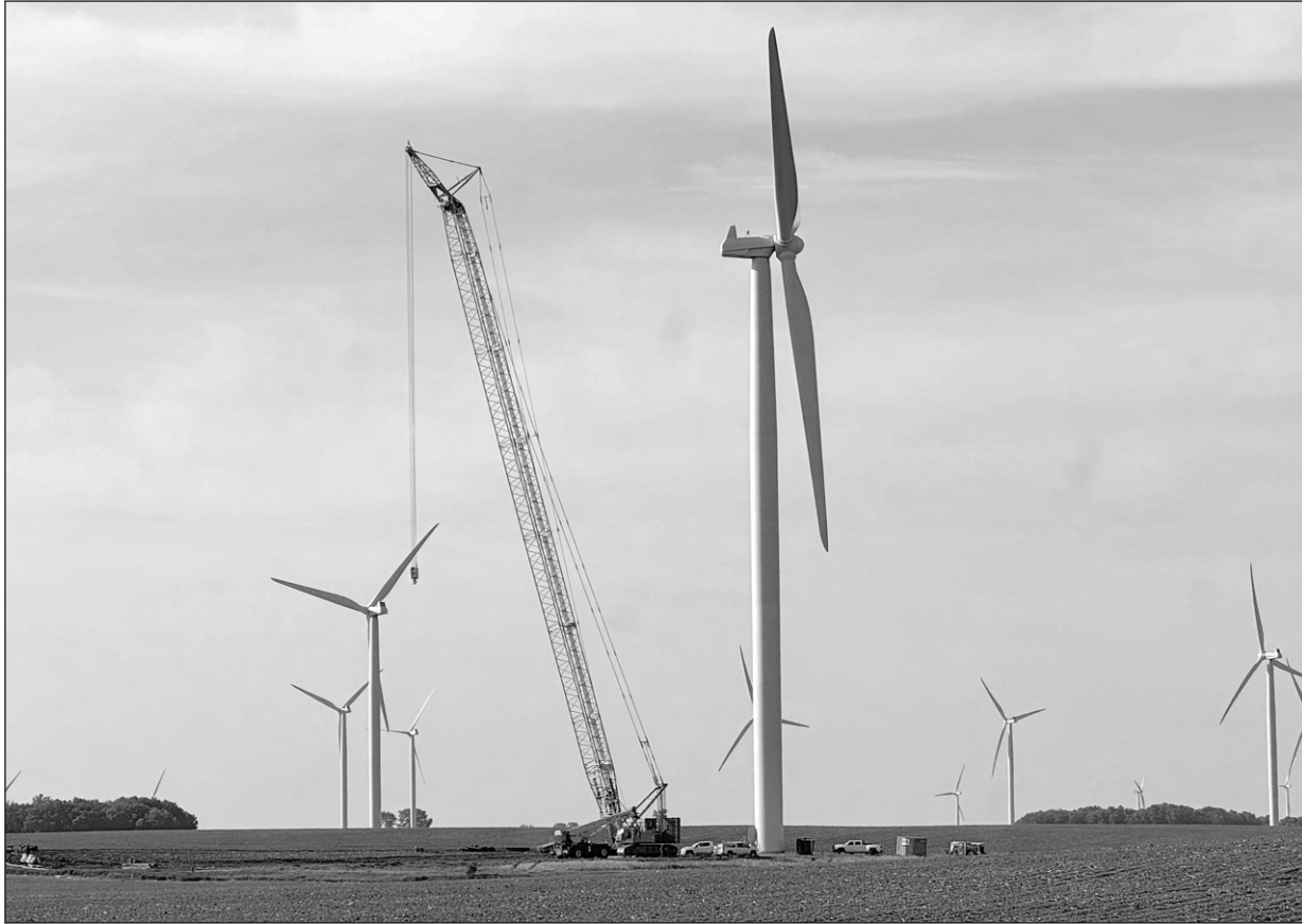
TOWERING REBUILD - A two-year project is underway to refurbish 122 wind turbines at Bent Tree Wind Farm located south of Hartland. Star Eagle photo by Deb Bentley
