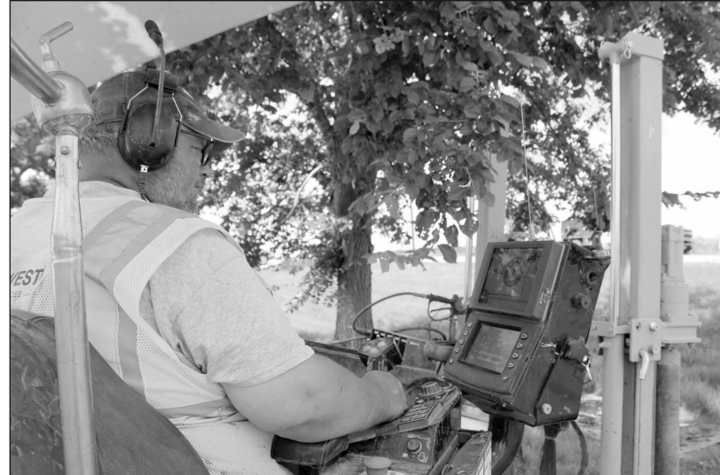
Above: Experienced operators of the directional borer say it can dig a channel up to a mile long. Below: Operator Scott Kroenke at the controls of the borer. Photos by Deb Bently
