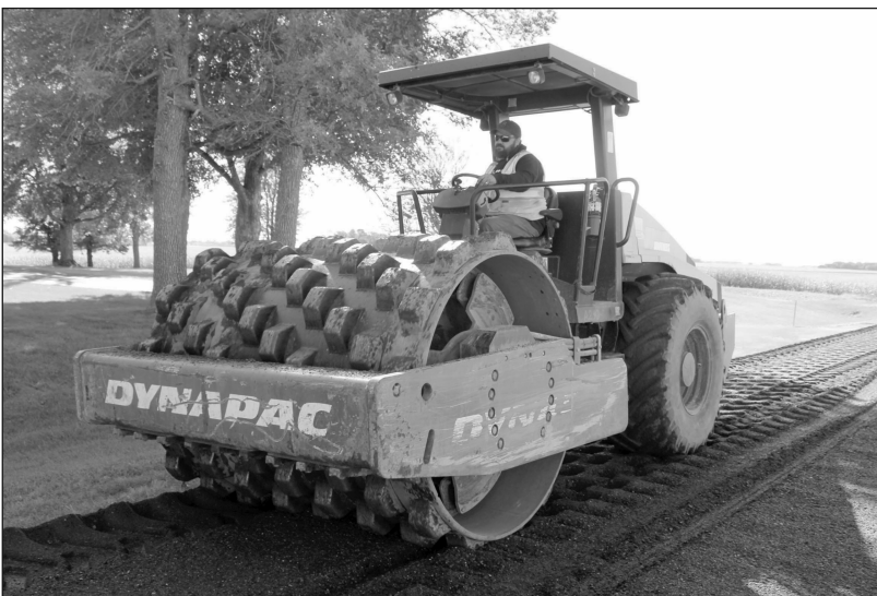
The “sheeps’ foot” compressor is the first machine to begin compacting the “reclaimed” asphalt after it has been lifted off of its former road bed. Star Eagle photo by Deb Bently
