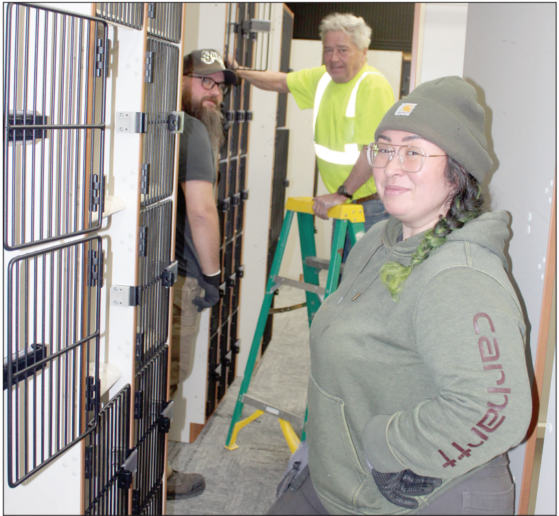
A four-person crew from Wengert of Owatonna spent two days in the NRHEG band room delivering, assembling, and facing 23 cabinets which have specialized space for musical instruments. Crew members included (from left) Jace Allen, David Riley and Kimberly Kwapick.
