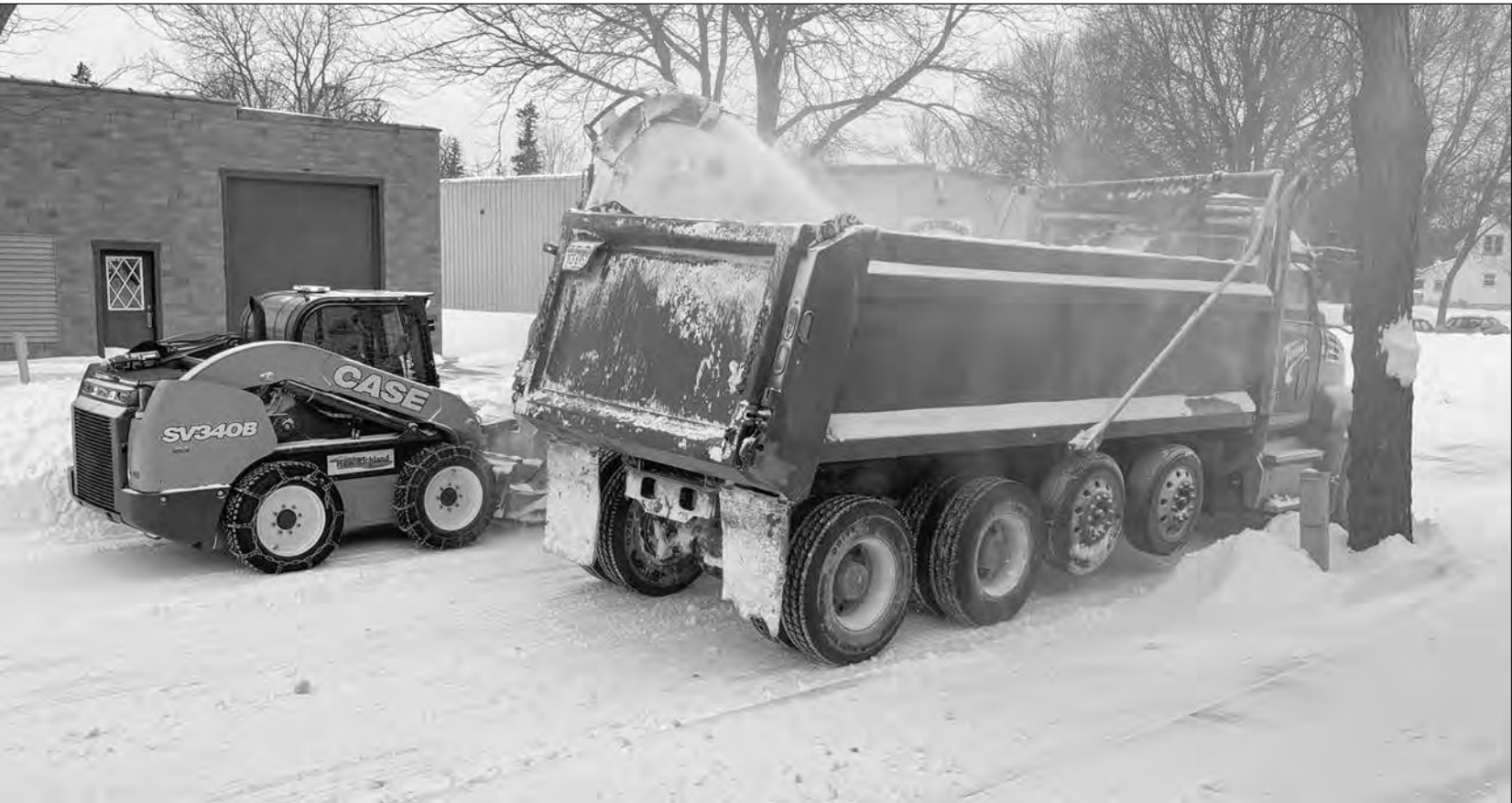
WORKING HARD - The City of New Richland recently thanked the City's Maintenance Crew on Facebook for working diligently to ensure the streets are clear for the residents to navigate. "We acknowledge that some of these piles are substantial and may be an inconvenience, but clearing Broadway alone has taken all day. Please be kind and patient while our crew members work hard to complete the task. This isn't a one day job."
