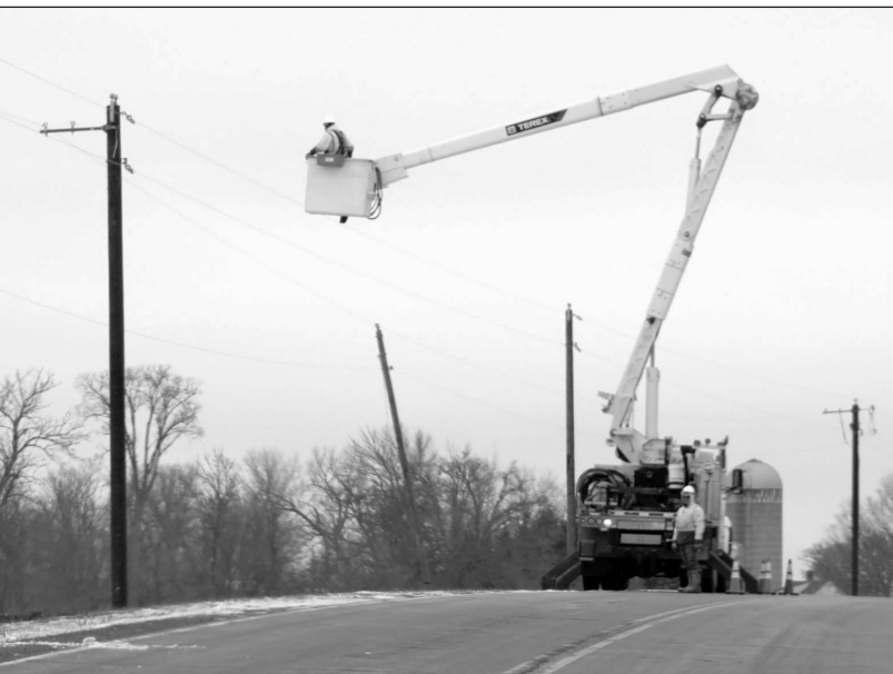
A Steele-Waseca crew in the process of replacing a Waseca County power line. The poles of the existing line have been set at an angle to allow the new poles to be installed.
